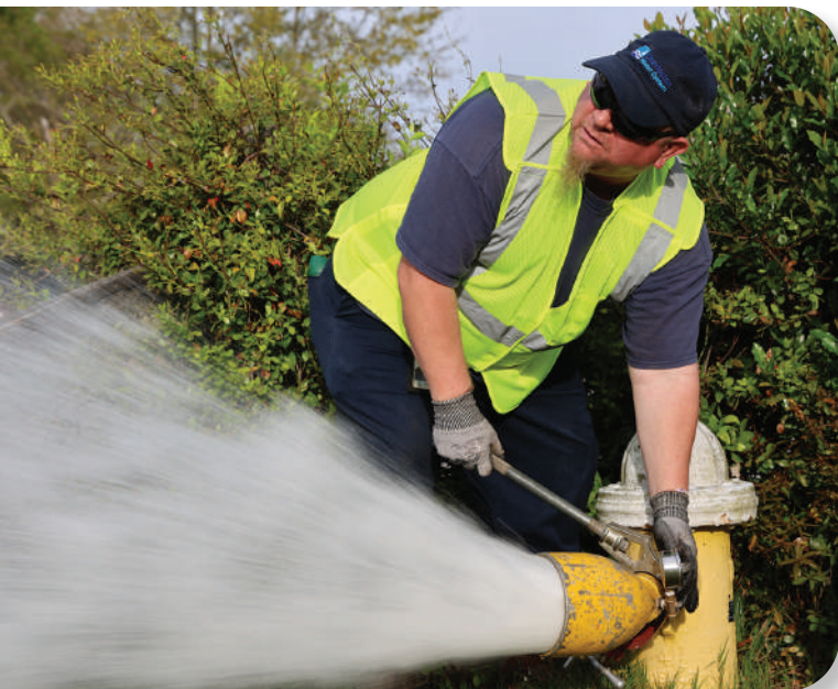
Hydrant Maintenance Operator Will Wade and his Water Distribution team members flush fire hydrants to support water quality and to help prevent discolored water.
